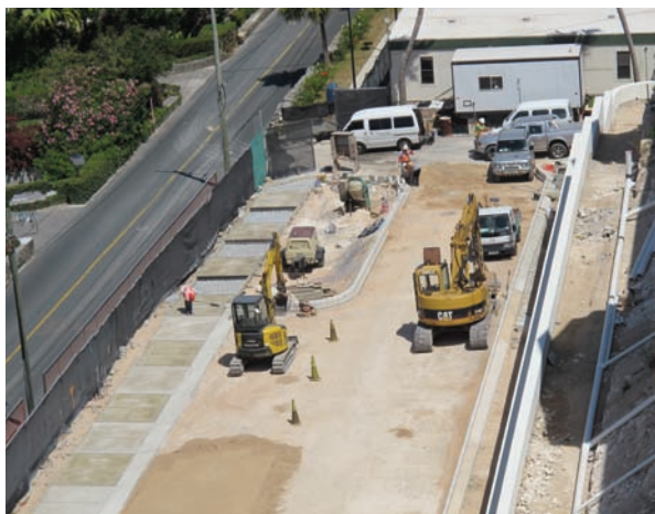
Aerial view of phase one of the Acute Care Wing entranceway.
