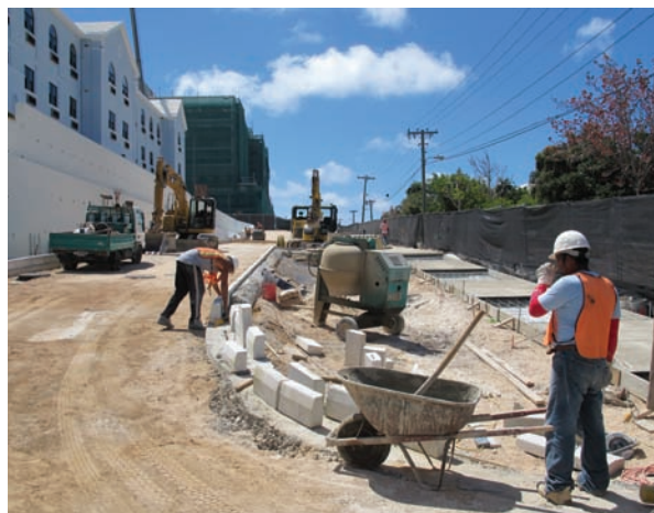
Phase one of entranceway works underway.
