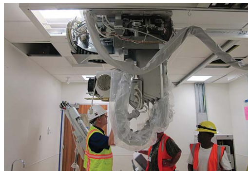
Installation of X-ray equipment - 15 May 2014
