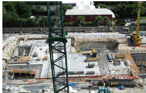
Roof slab on the sewage treatment plant almost complete.
