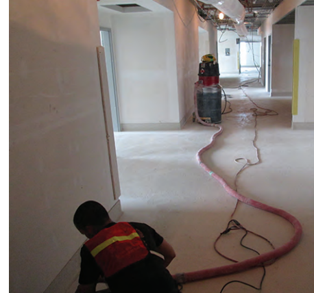
Terrazzo flooring works underway.
