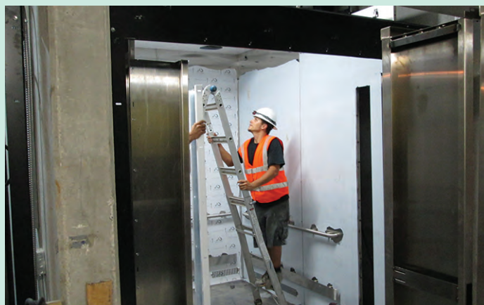
Elevator fitting works underway.
