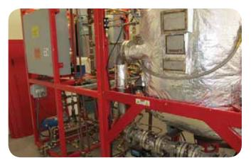
As BHB manages medical waste for the entire island, the new system was a required investment for Bermuda as well as the hospitals. Two macerators were therefore installed to ensure medical waste will not build up if one requires maintenance. The new macerators also resulted in significant savings.
