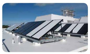
Twenty-four solar panels on the roof would pre-heat water for the inpatient room floors, saving around 9,000 gallons of fuel per year, and renewable energy ensured hot water would be available around the clock.
